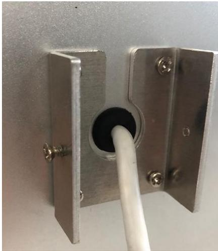
9. Hang the bracket on the back of the machine on the bracket fixed on the wall, as shown below.
